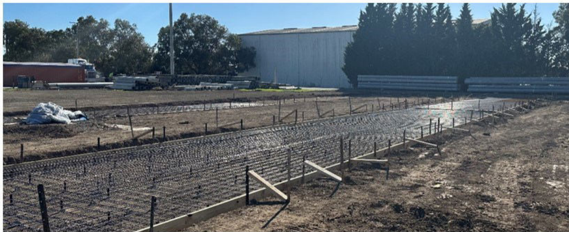
Progress photos of construction underway, with project completion well in sight
