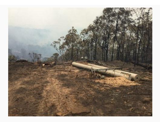
A perfect example above of *Build Back Better* with two Titan HV transmission poles ready to replace the bushfire destroyed poles that represented the original risk – which is now to be eliminated.
