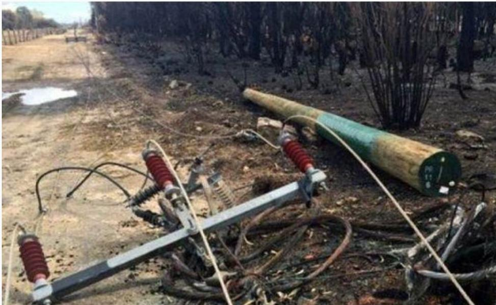
The intention in this fire prone area appears to be to reintroduce this risk factor into the network, by reinstalling another wood pole supporting crucial operational equipment.
