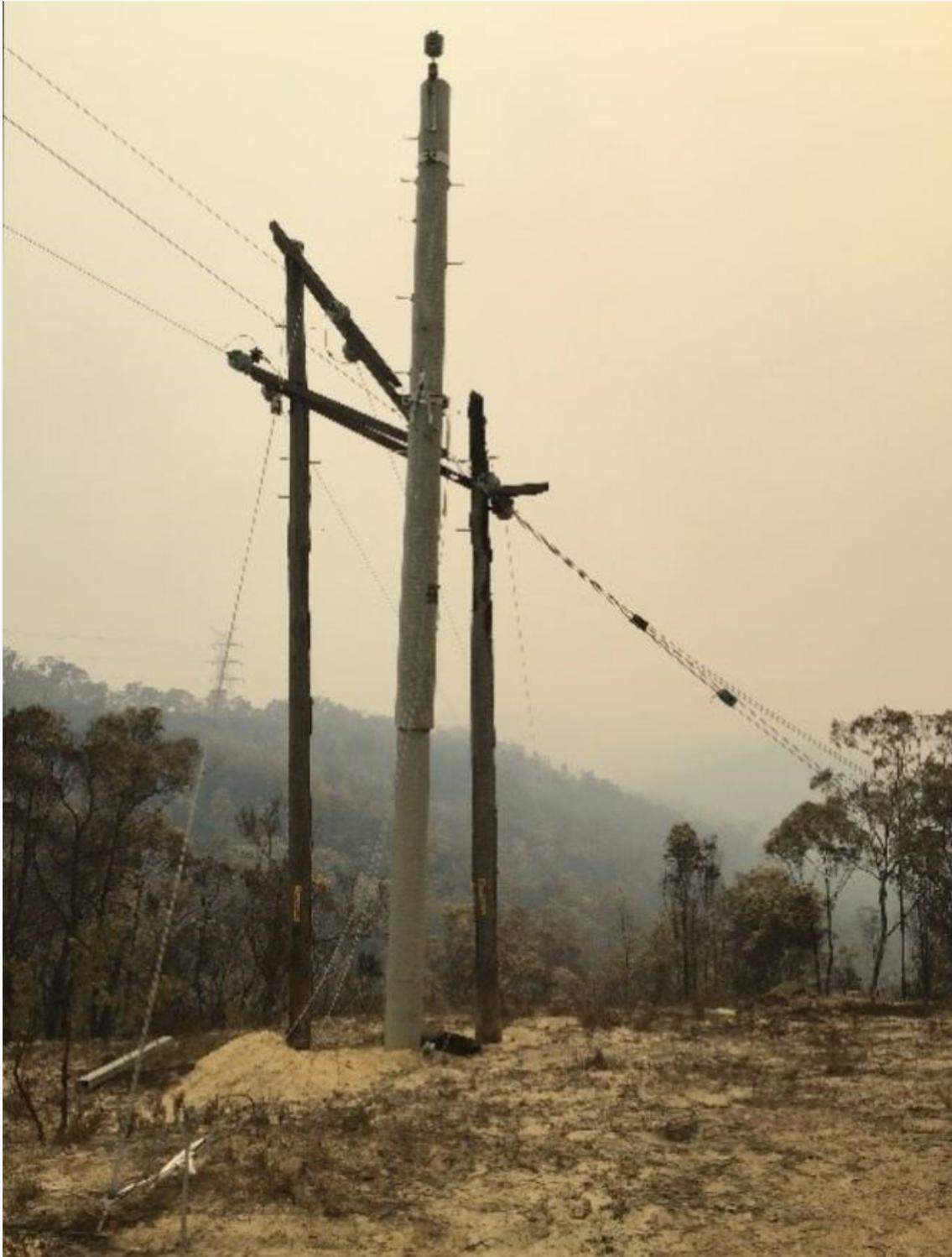
Introducing durability into the network with a 2 part bushfire proof Titan replacing fire destroyed timber poles in a fire prone area. A perfect example of the United Nations, Build Back Better policy
