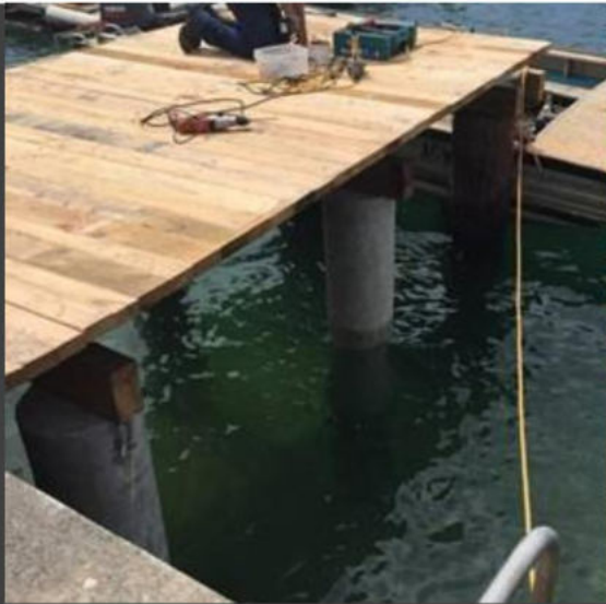
Wharf under construction with Titan foundations
