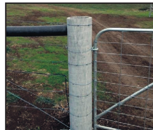
Detail of gate attachment to a Titan Post.
